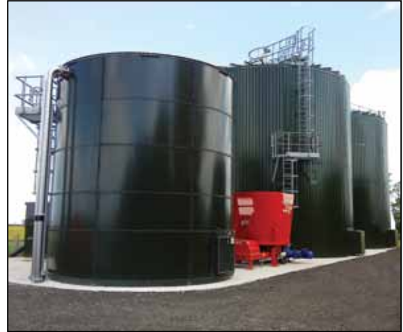
Anaerobic Digester
