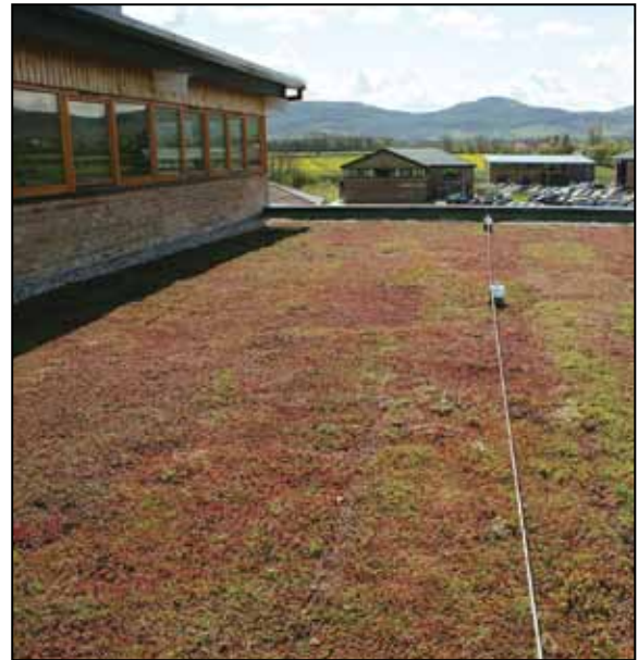
Green Roof at Momentum Business Centre
