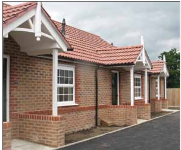
Oxmoor Place development at Easingwold (Yorkshire Housing)
