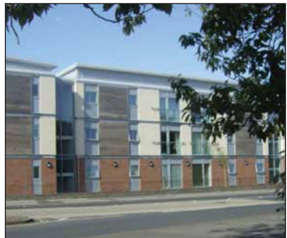
York Vale House development in Northallerton (Broadacres)
