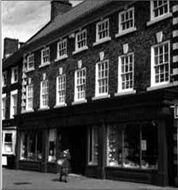
102 High Street, Northallerton
